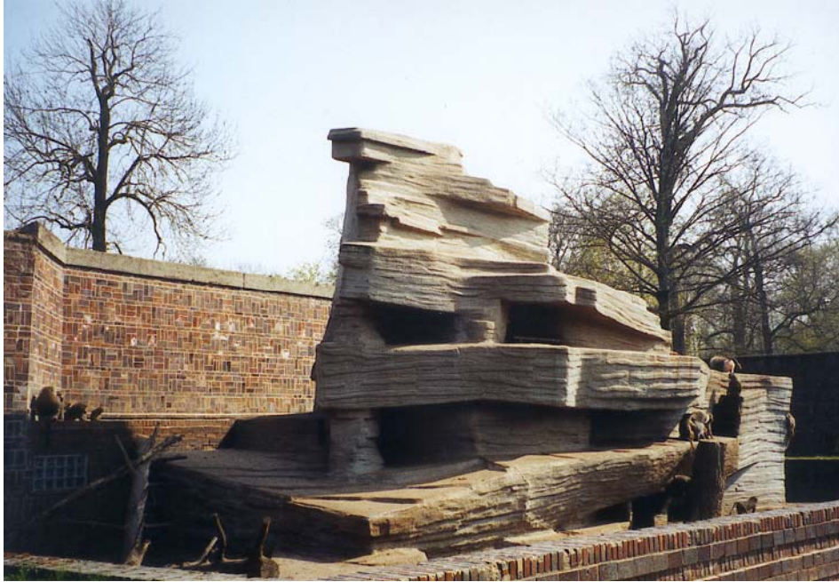
Figure 2.3 b The baboon facility seen from the left side
